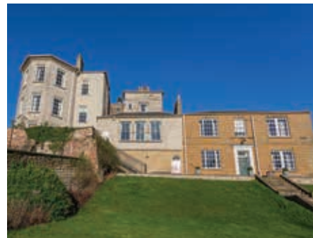
The Talbot viewed from the river side, with on the right the former private house called The Cloisters, now a bedroom wing of the hotel.
