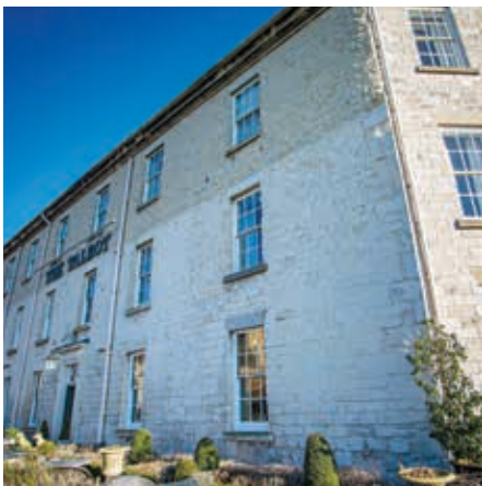
A view of the west-facing elevation of The Talbot reveals the changes in brickwork marking the extension, probably constructed shortly after 1767, and the third storey added in 1808/09.
