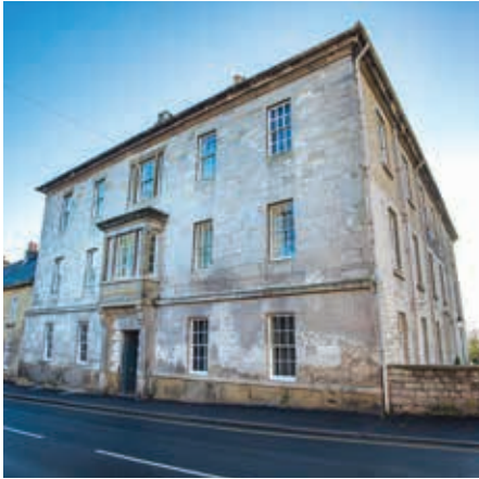
The street elevation of The Talbot Inn, seen today exactly as it looked after the rebuilding work in 1809, which included a third storey and the addition of an oriel window above the street-side entrance.
